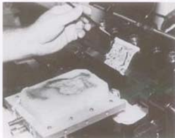
Fig 4. — Using a motorized sledge microtome, complete sections of long bones, joints, and bone tumors are prepared in the Orthopedic Histology Laboratory.
